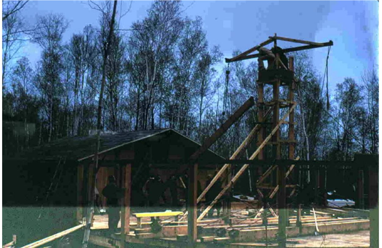
Hoisting first rafter
